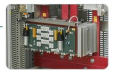
Galvanic insulation boards generate and provide information for analysis of the power diodes state diagnostics system with controller.
