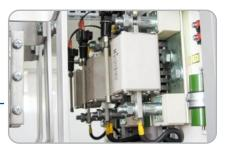
Protection of power semiconductor devices (diodes) against internal and external switching surges is implemented in rectifiers. Each diode is protected against internal switching surges with RC circuit, installed on the galvanic insulation board, and against external switching surges combined with RC circuits and variable resistor with fuses, installed on the switching surges protection panels.
